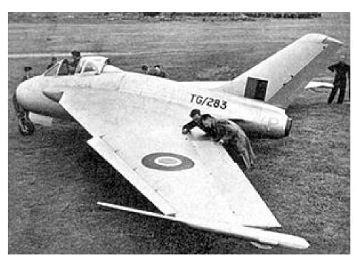
The de Havilland DH 108 "Swallow" was a British experimental aircraft designed by John Carver Meadows Frost in October 1945. The DH 108 featured a tailless, swept wing with a single vertical stabilizer, similar to the layout of the wartime German Messerschmitt Me 163 Komet rocket-powered point-defense interceptor. RAF Capt. Eric Brown (now deceased) flew it after the first prototype crashed attempting to break the sound barrier.
