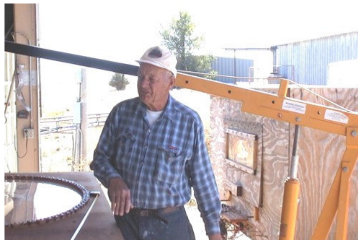
Here's George explaining a little about the entire process of forming a new canopy. The hoist will raise the panel and allow it to be flipped over. The short loops noted in a previous picture will then allow the hoist to raise the panel up to the height of the heat box and put it in place. I am sure this saves a lot of back aches.
