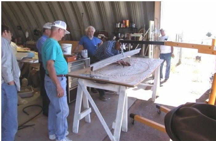
Now you can see the panel flipped over and the short cable hooked up for the hoist to the top of the box. George is installing the air pressure fitting into the hole that will eventually blow the canopy and provide a source for the pressure gauge.
