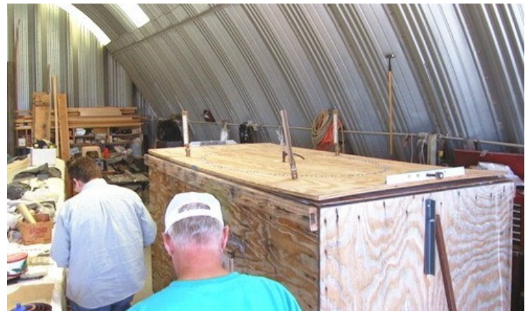
The panel is now on top of the heat box. It is secured at the four corners with wood screws which is sufficient to seal it from loosing very much heat. You can see the three thermometers sticking out of the panel on the left and right of the box. He records temperatures every 5-minutes until reaching the desired level evenly distributed throughout the interior which is lined with fiberglass insulation.
