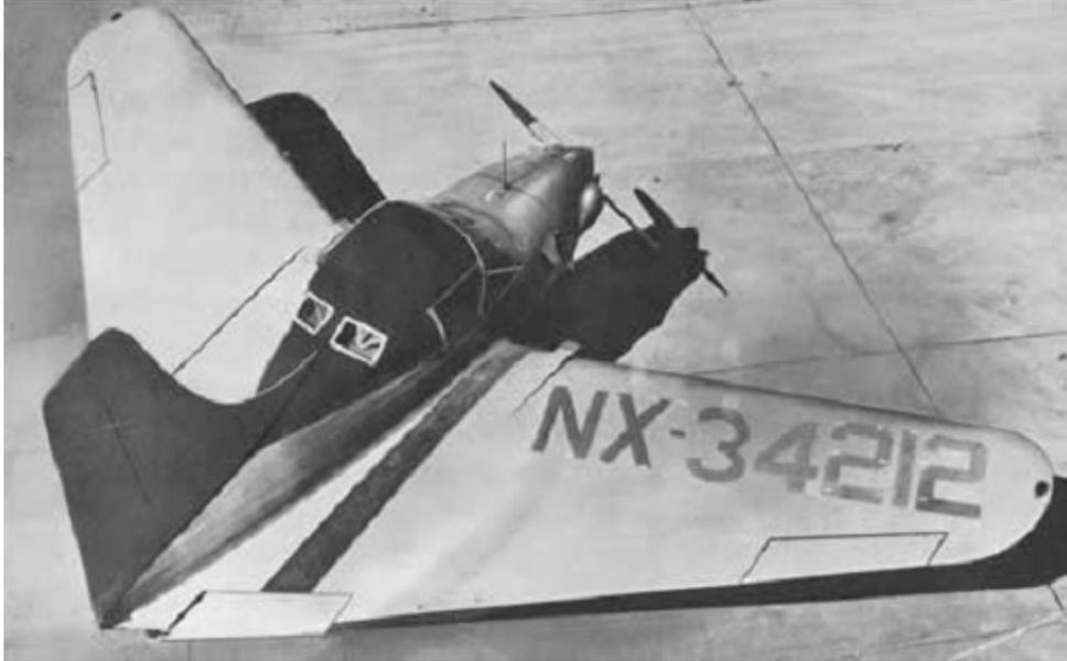
George Cornelius of Dayton, Ohio, was a staunch advocate of the swept-forward wing concept, which lent itself well to this experimental tailless aircraft (Mallard above) of the 1940s. Cornelius claimed that the combination of variable incidence wing and forward sweep resulted in an aircraft that was virtually stall-and spin-proof. Source: [http://www.century-of-flight.net/Aviation\\_history/flying\\_wings/usa.htm](http://www.century-of-flight.net/Aviation_history/flying_wings/usa.htm)
