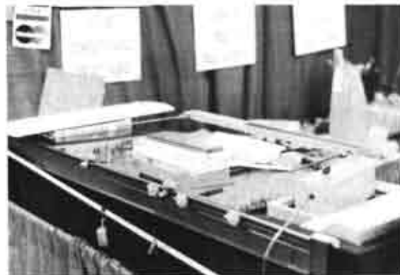
View of swing arm and linkage of "Feather Cut". Weights on bow arms are adjustable for top and bottom cuts.
