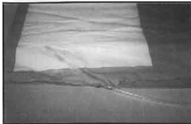
Photo 1 - Sealed end of vacuum bag. Note that the vacuum line is well into the bag, and that the end of the vacuum line is onto the breather cloth. This stops the vacuum bag from sealing off the end of the vacuum line before the vacuum is removed from the bag.
