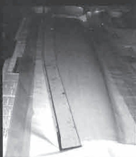
Iron bars are used to insure a nice, straight trailing edge.
