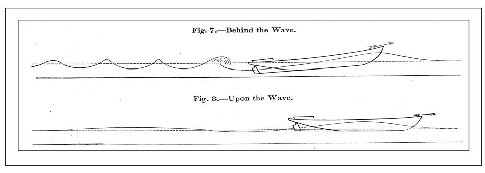
Figure 23: Russell's 1839 sketches of a canal boat towed at speeds less than and greater than the speed of its solitary wave.
