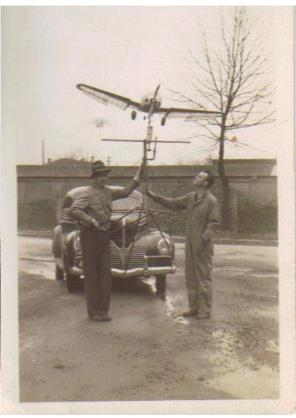
Mallard model in skeleton form and covered and attached to a fixture mounted to an automobile as an "open range" wind tunnel.
