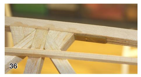
There is also a 0.025" brass pad on the underside of the top fuselage longeron that is 1/4" X 7/8". Note this pad has a small dimple that keeps the latch from rotating forward on its own, once it is in the closed position.
