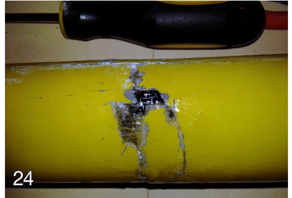
24. Put a little extra epoxy in the big holes. (I had dripped in some extra epoxy before running the cloth in also.)
