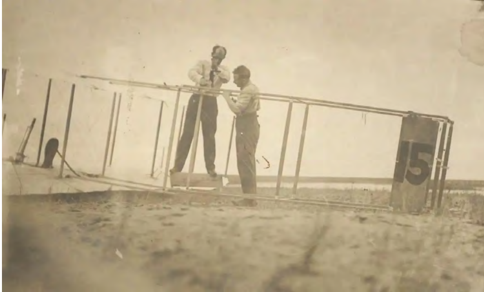
Extending the tail, note the hand-drill that Orville (left) is using. (credit: Photo: Joyner Library)
